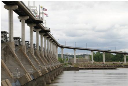
▲ There are 18 locks and dams – 13 in Arkansas and 5 in Oklahoma; each lock chamber is 110' wide x 600' long and can handle an 8-barge tow.
